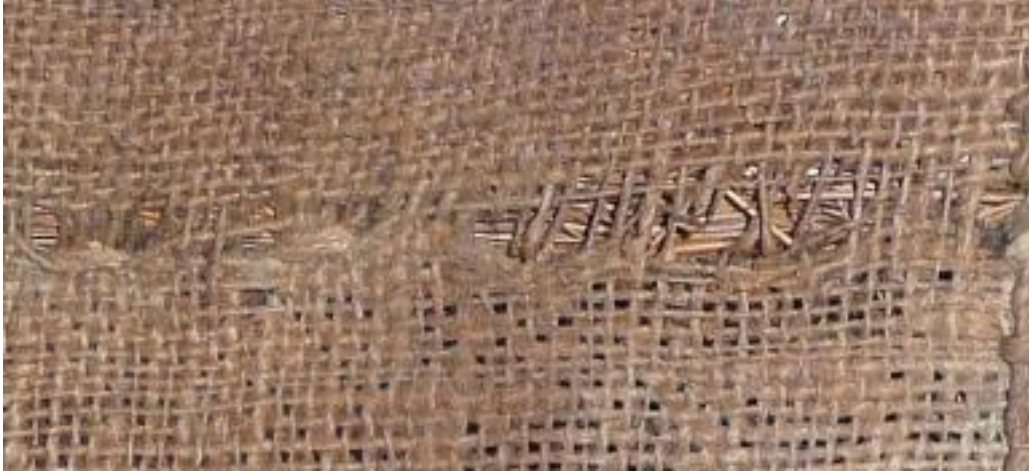
Figure 21: Detail of figure 19. The marsh grass stuffing is visible through a tear in the sackcloth on the underside of the seat.
