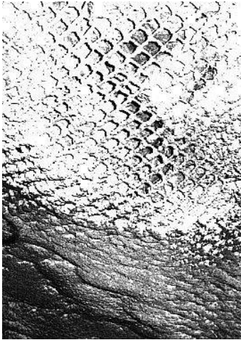
Chainlink mesh, while very strong and flexible, is not ideal for shotcrete application because it is difficult for the shotcrete to penetrate the mesh.
