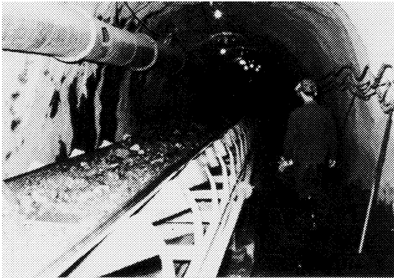
Figure 11.2: A conveyor tunnel with grouted rockbolts and shotcrete support. Here the tunnel has been designed for a life of about ten years and possible corrosion of the support system was a major factor in the choice of the support.
