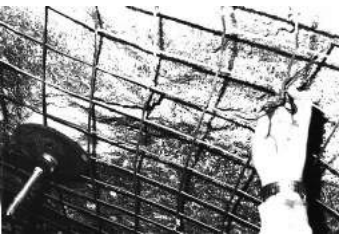
Welded wire mesh, firmly attached to the rock surface, provides excellent reinforcement for shotcrete.
