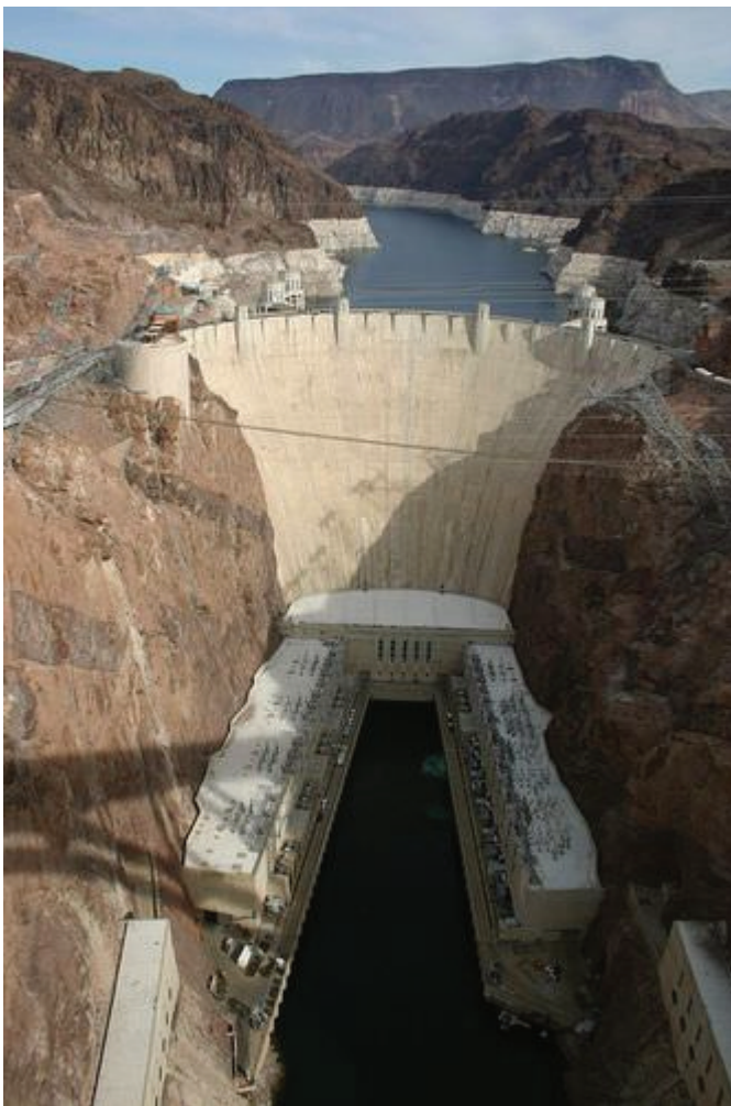
Figure 3. Hoover Dam, Nevada, U.S. Hoover Dam, Nevada, U.S.. Behind the dam is Lake Mead, the largest reservoir in U.S.. White band reflects the lowered water levels in the reservoir due to drought conditions from 2000 – 2010. Source: Cygnusloop99 at Wikimedia Commons
