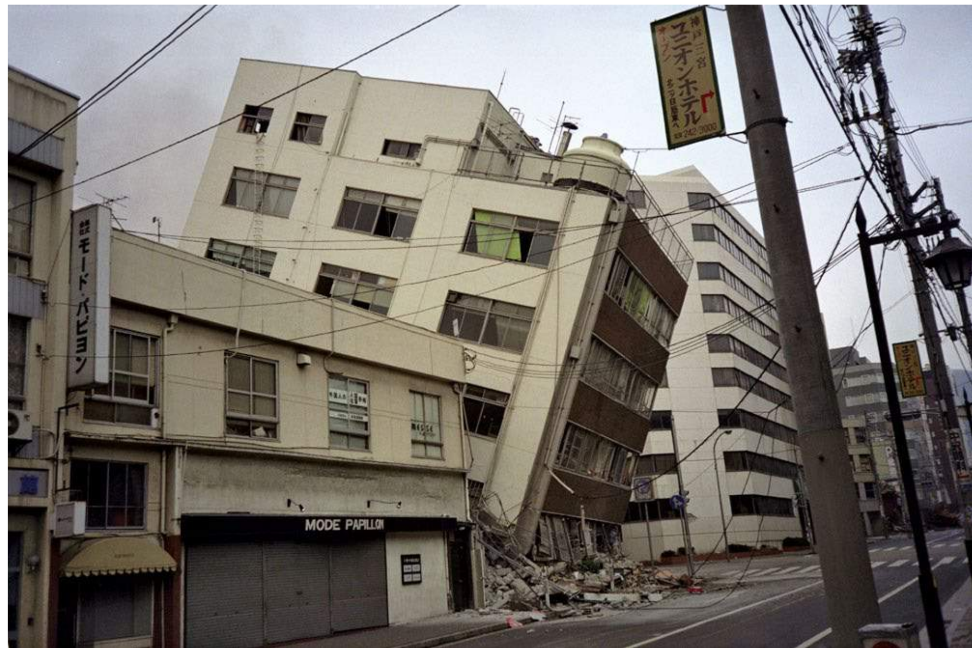
Collapse of a building due to earthquake
