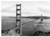
1. Cables and Arches
