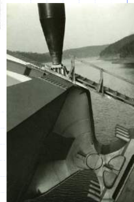
The bearing of the arch
