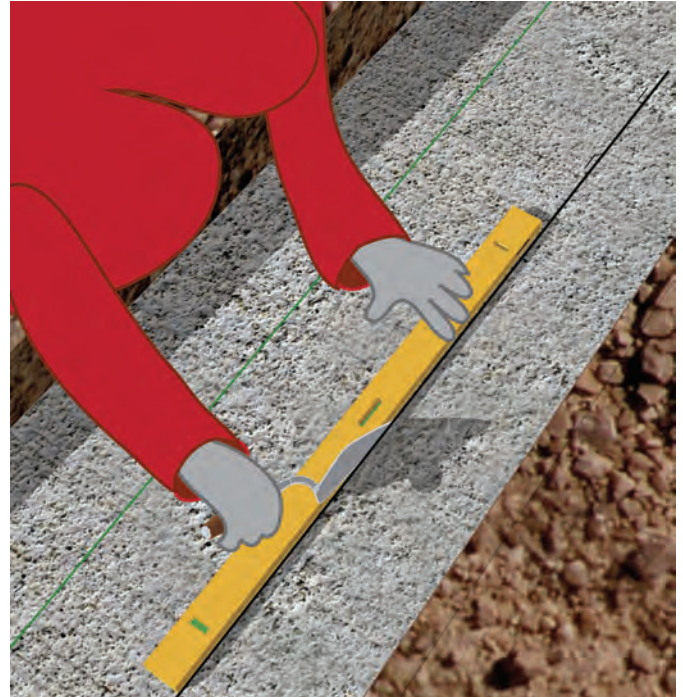
11.11 - After a second line is transferred down a little further along, the lines are joined using a level or straight edge.
