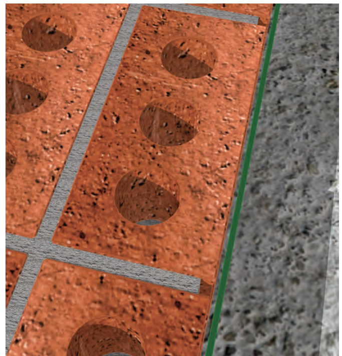
11.16 - Bricks are laid next to, but not touching the line, otherwise the line may be pushed out of position and the wall will not be built straight.
