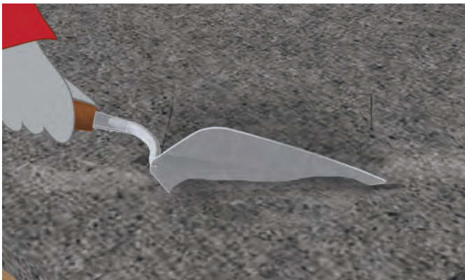
11.5 - Mortar for the bed is picked up with a sideways motion of the trowel. The trowel should be filled with mortar then lifted and the mortar deposited firmly in position.
