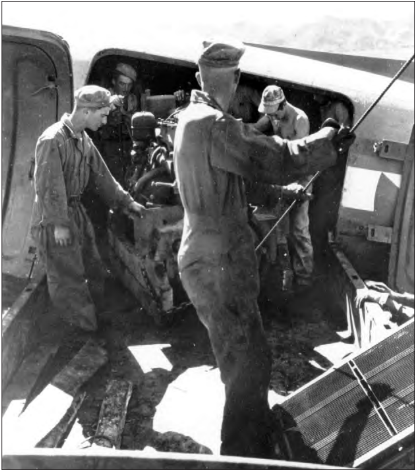
Engineers unload a bulldozer from an Allied transport plane. (U.S. Army Military History Institute)
