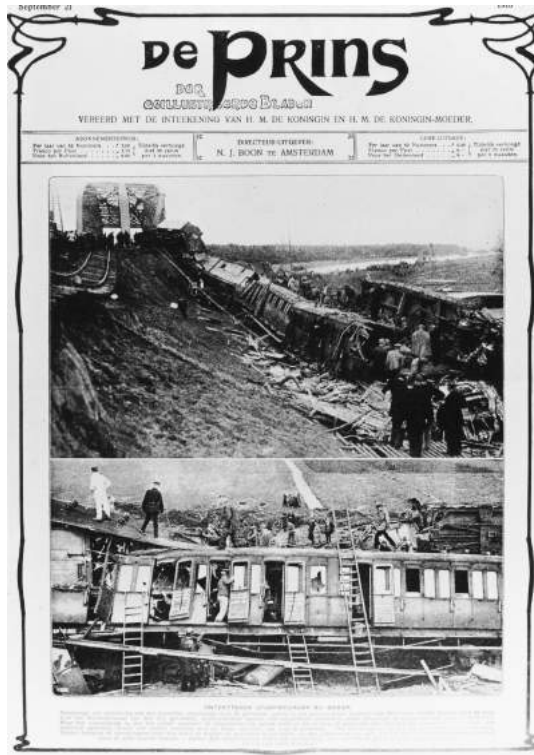
Figure 1.1: Landslide near Weesp, 1918.
