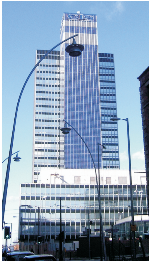
Fig. 8. The CIS Tower, Manchester, England, was clad in PV panels at a cost of £5.5 million. It started feeding electricity to the national grid in November 2005. Credit, Pit-yacker.
