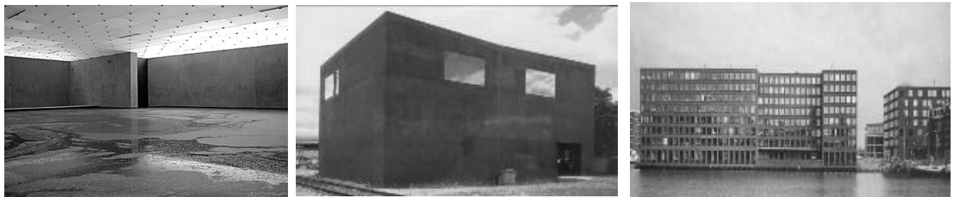
Figure 9. Peter Zumthor: Kunsthaus, Bregenz, Switzerland, 1997. / Figure 10. Gigon&Guyer: Switching Station, Zurich, Switzerland, 1996-99. / Figure 11. Diener & Diener: KNSM - and Java - Island Apartment Blocks, Amsterdam, The Netherlands, 1995-2001.
