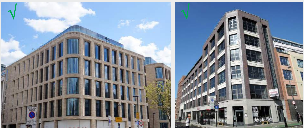
Figure 10 Emphasising junctions. Corners are often best addressed by creative articulation rather than any height increase. The Turnmill Building (top) and John Jones (bottom) show both an appropriate corner treatment with curved facade/wrapped fenestration and good rhythm, scale and proportions. Even though the buildings have relatively large footprints they do not appear out of scale with their surroundings due to vertical proportioning.
