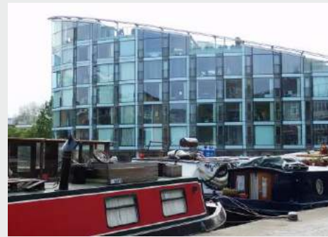
City Road Basin
