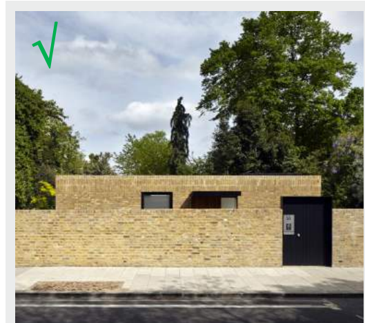
Figure 21 Gap infill development. This successful development appears as part of the existing front wall. This approach retains the boundary wall and of the corner property and views into the rear gardens which are an important feature of this conservation area.
