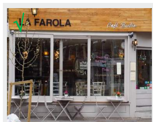
Figure 34 An approach to designing an openable shopfront which successfully maintains an appropriate solid to void ratio.
