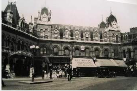
Highbury Station as originally built
