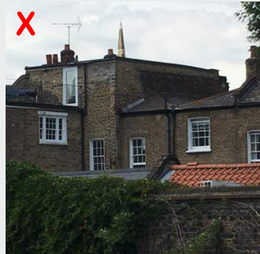
Figure 22 The roof extensions in the top image have been designed in a style appropriate to the host buildings and to maintain the prevailing roofline. In contrast, the roof extension in the bottom image projects significantly above the prevailing roofline and its size and treatment does not respect the scale and form of the host building or the rhythm of the wider terrace.
