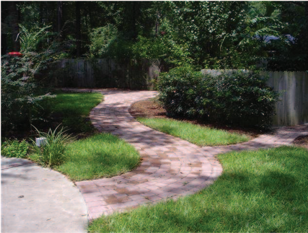
Figure 26. Permeable walks, such as this paver brick path installed on compacted base material, will allow rainwater to filter through or around the paved surface. These pathways can also make previously unreachable areas accessible to wheelchairs or strollers. Photo by Pat Drackett. Landscape contractor: GroundScape Inc., Biloxi.
