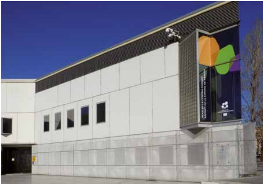
Facade of the Archive’s premises in Almogàvers St., opened in 1993. On it appears the insignia of the European Heritage Label, granted to the Archives in 2015.
