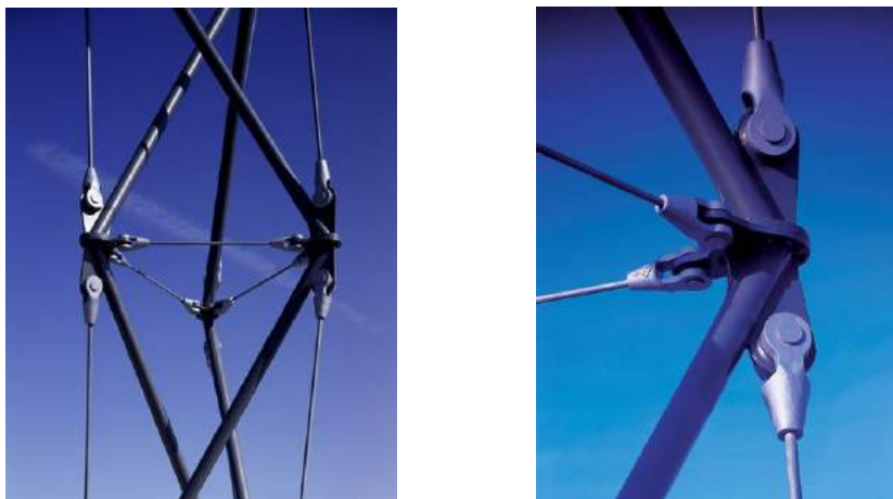
Figure 8.3.7: Warnow Tower- Assembly of twist elements and node details ©Mero
