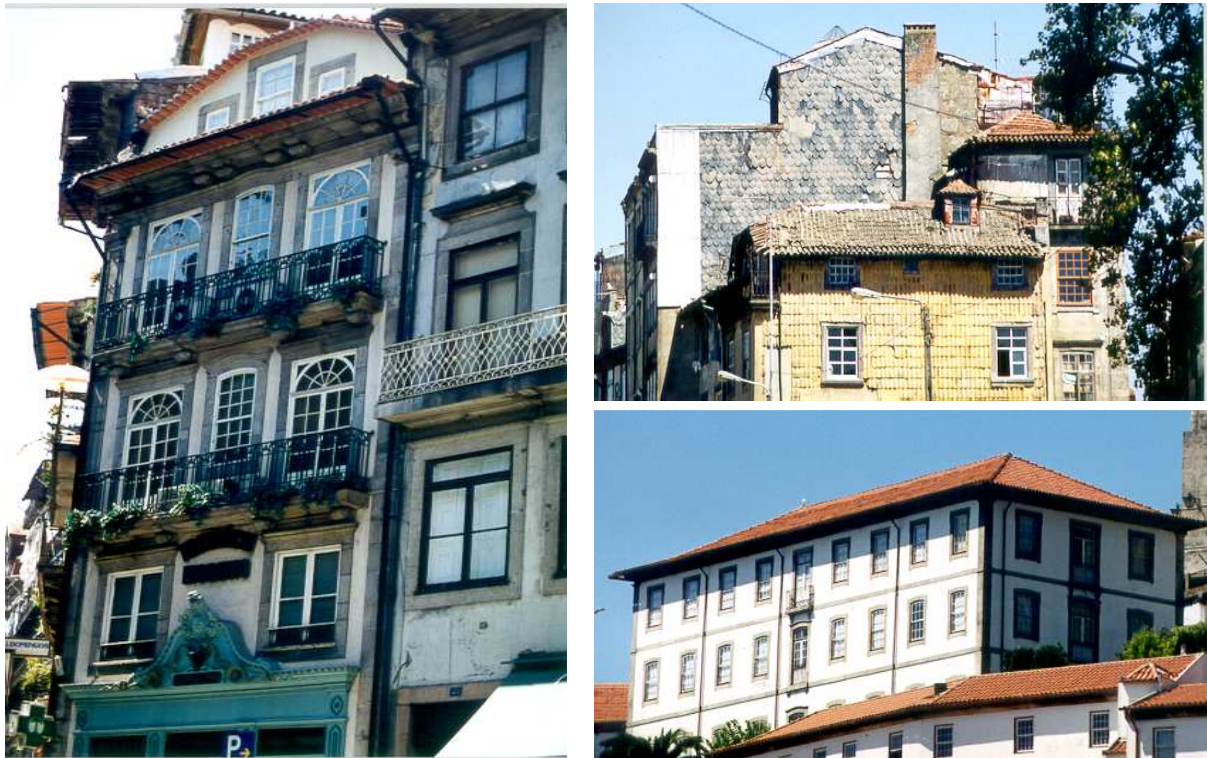
Figure 3: Examples of some Portuguese traditional buildings
