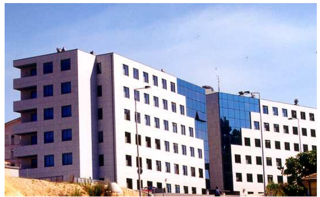
Granite stone tiles
