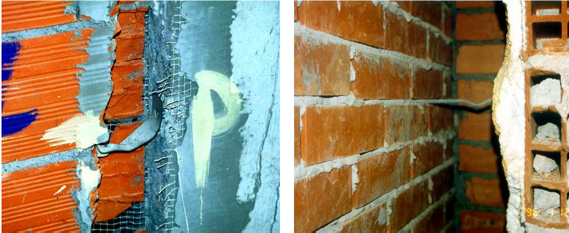
Figure 8: Examples of some ties and anchors used in Portugal
