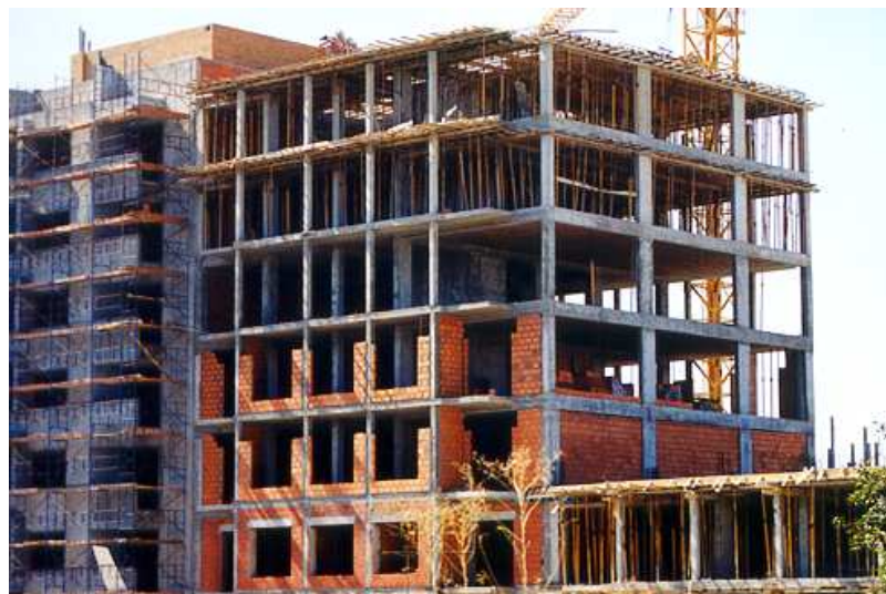
Figure 2: Example of typical buildings with reinforced concrete frame structure
