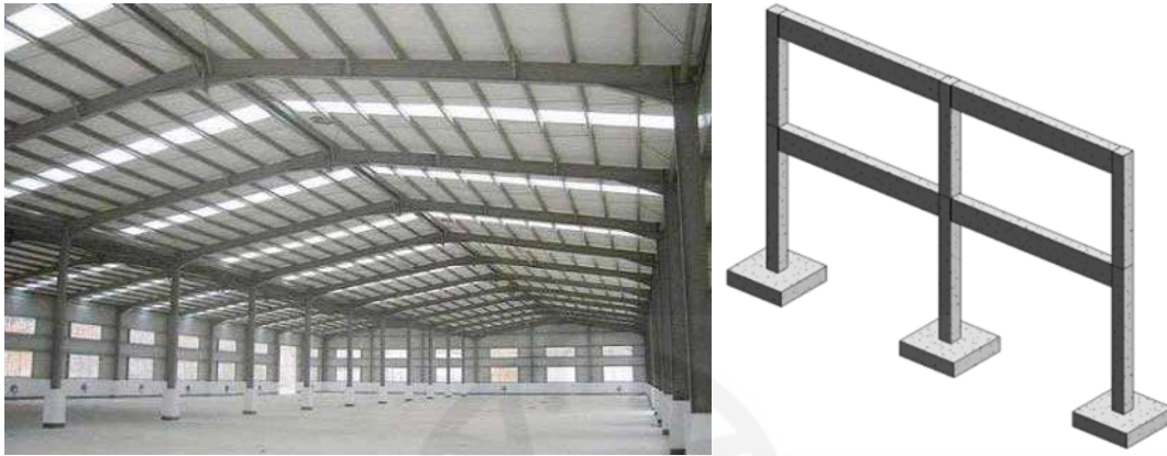
Figure 1-7: Steel and concrete frames
