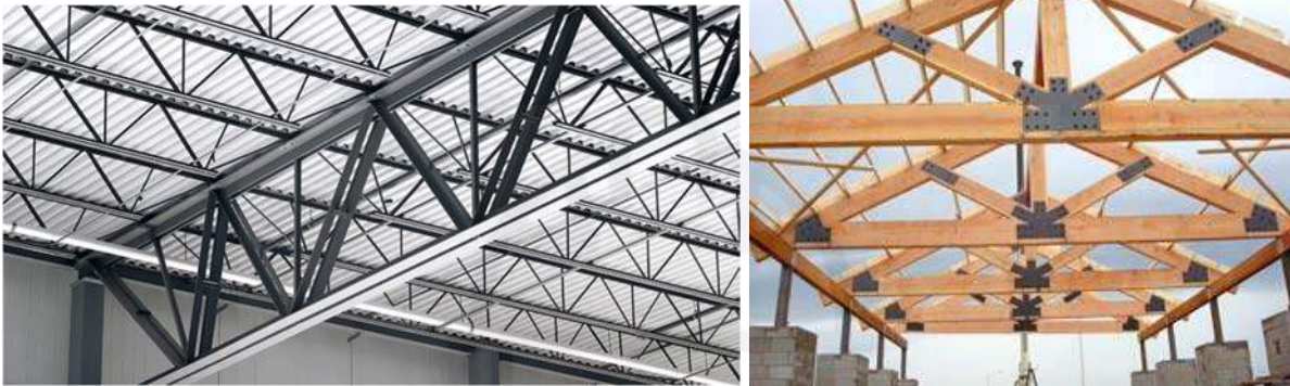
Figure 1-5: Steel and timber trusses
