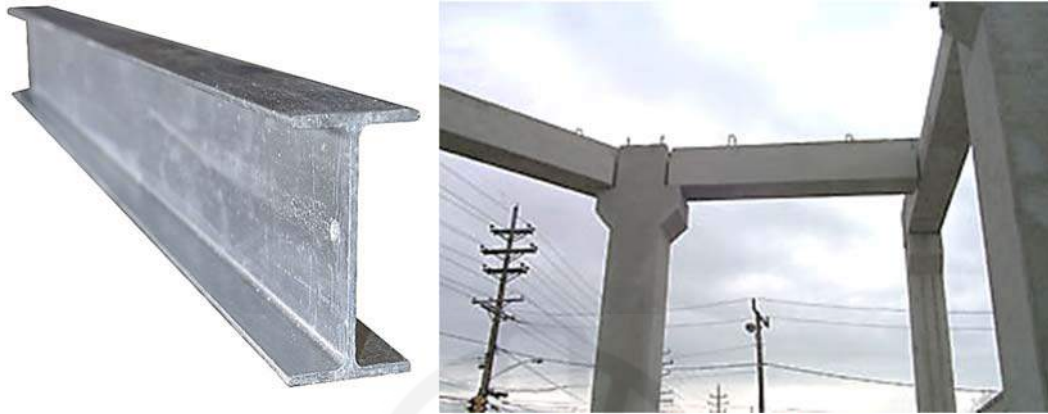
Figure 1-3: Steel and concrete beams
