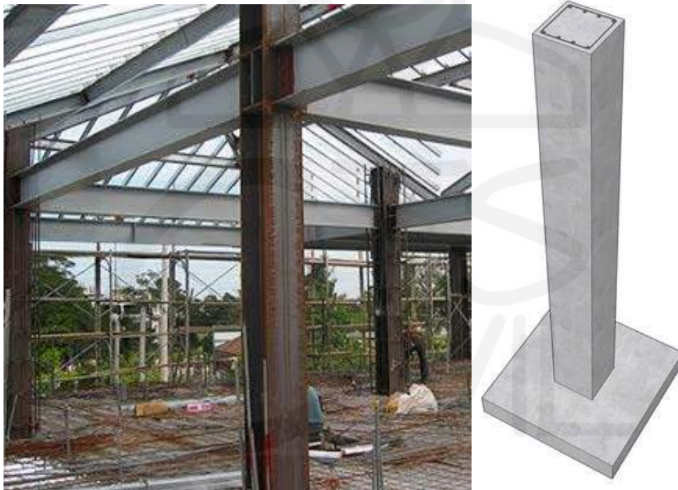
Figure 1-4: Steel and concrete columns
