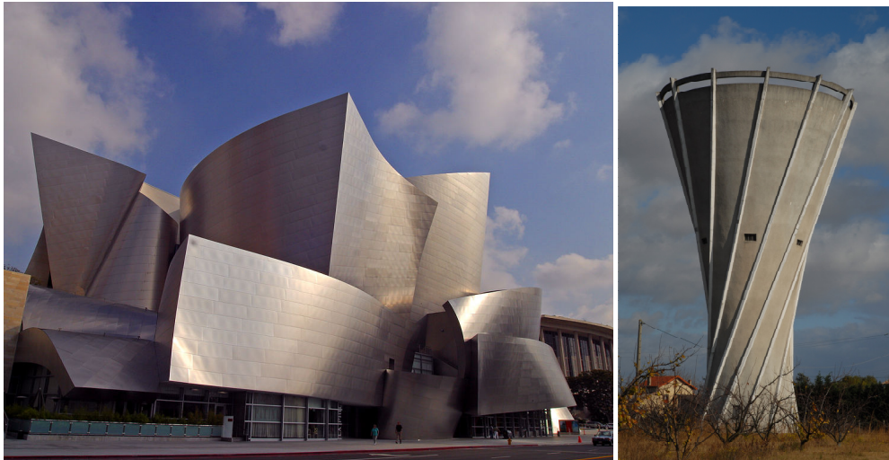
Figure 10: Two usages of particular curved surfaces. Left: The Los Angeles Walt Disney Concert Hall with a stainless steel façade, piece-wise developable, image by J. Sullivan (2004), courtesy of PDPPhoto.org. Right: Water tower in La-Roche-de-Glun (France), with a one-sheet hyperboloid ruled surface; image by A. Rambaud (2007), with permission
