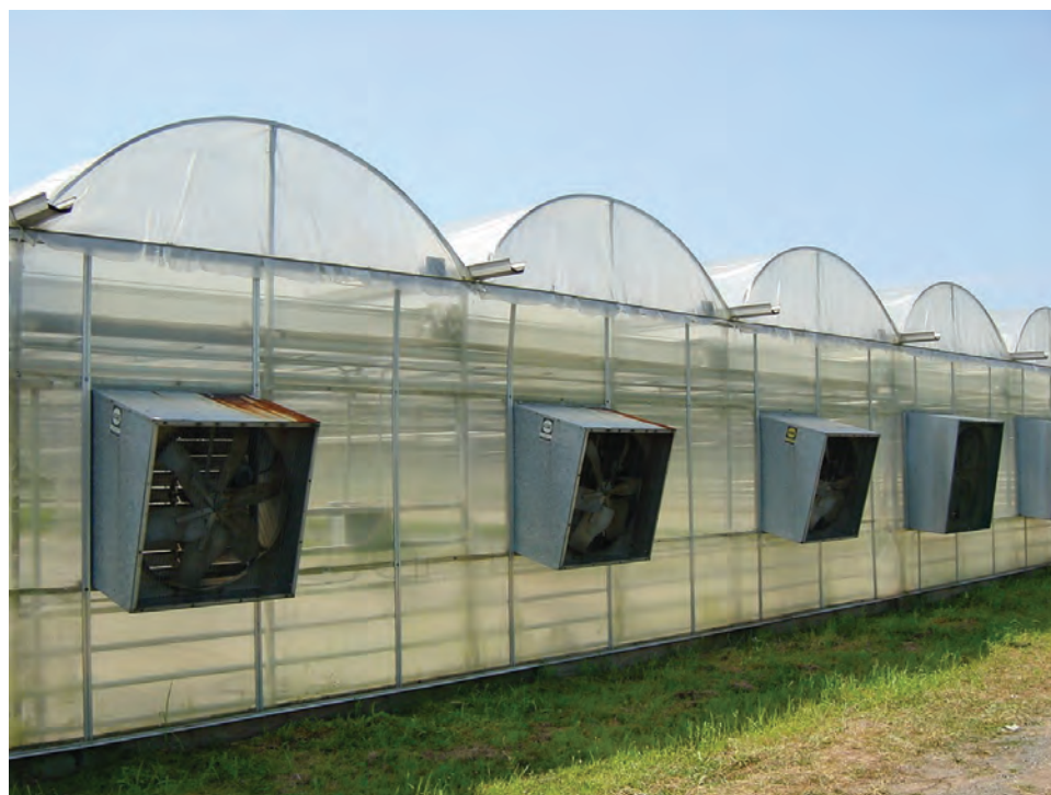
Figure 3. Gutter-connected greenhouses with mechanical ventilation. (Photo by A. J. Both)
