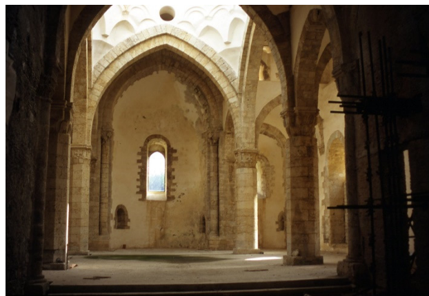
Figure 3. Church of Santa Maria della Valle (called Badiazza), central apse. Image courtesy of https://www.cistercensi.info/abbazie/abbazie.php?ab=1165 (accessed on 20 May 2021).
