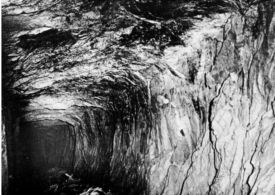
Figure 10a. Square tunnel in quartzite remote from mining activities. Depth of 9,500 ft. below surface in a South African gold mine
