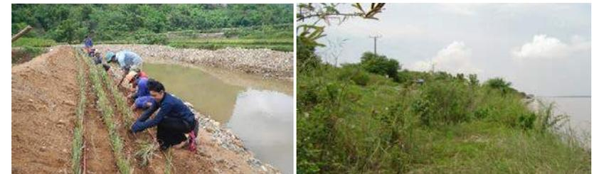
**Riverbank stabilization.** Vetiver grass planted along a riverside in northern Viet Nam (left) and the grassed flood foreshore with small trees on an embankment in Cambodia (right) provide for riverbank stabilization (photos by the International Centre for Environmental Management and J. Howell).
