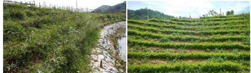
**Strongly rooted plants.** In northern Viet Nam, the method adopted of propagating shrubs and small trees for shallow stabilization of unconsolidated slopes is one that makes the plants produce a mass of fine, strong roots, which provide soil reinforcement. (photos by the International Centre for Environmental Management).
