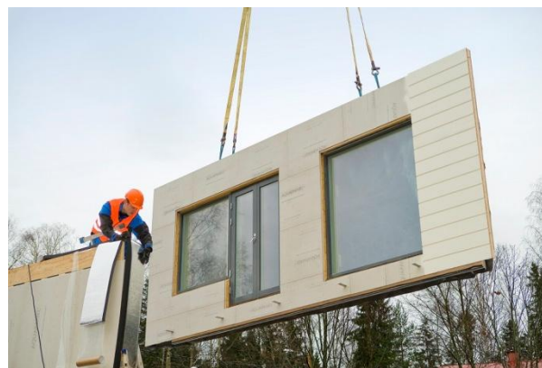
Figure 8 – Assembling of a prefabricated wall element.
