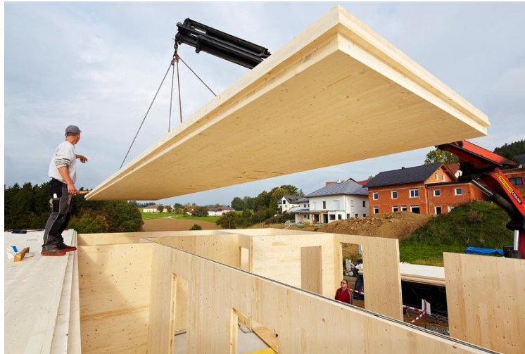
Figure 4 – Erection of one family CLT house in Austria.
