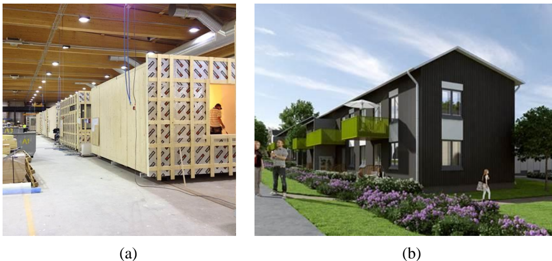
Figure 9 – Stora Enso Hartola CLT modules; (a) Modules pre-fabricated at the Hartola unit; (b) Ikea BoKlok multi-family modular CLT housing units in Vantaa.
