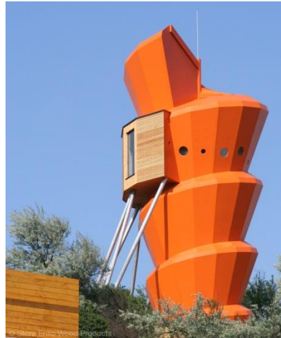
Figure 12 – Spiral Tower pre-fabricated with CLT.
