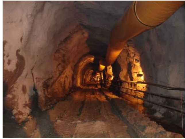
Fig. 2: Photograph showing Head Race Tunnel of Singoli-Bhatwari Project, Rudraprayag
