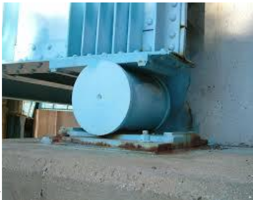
Fig. 2 Roller support
