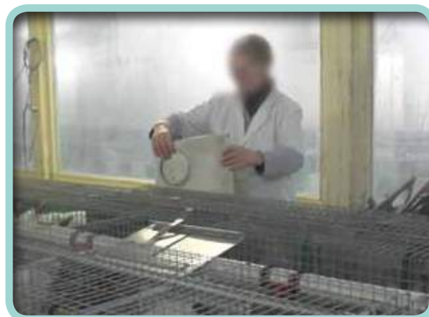
Installation des cloisons.
