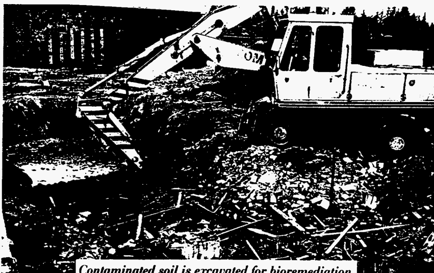
Contaminated soil is excavated for bioremediation
