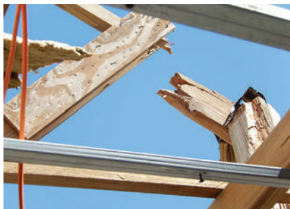
Figure 2 : Section insuffisante
