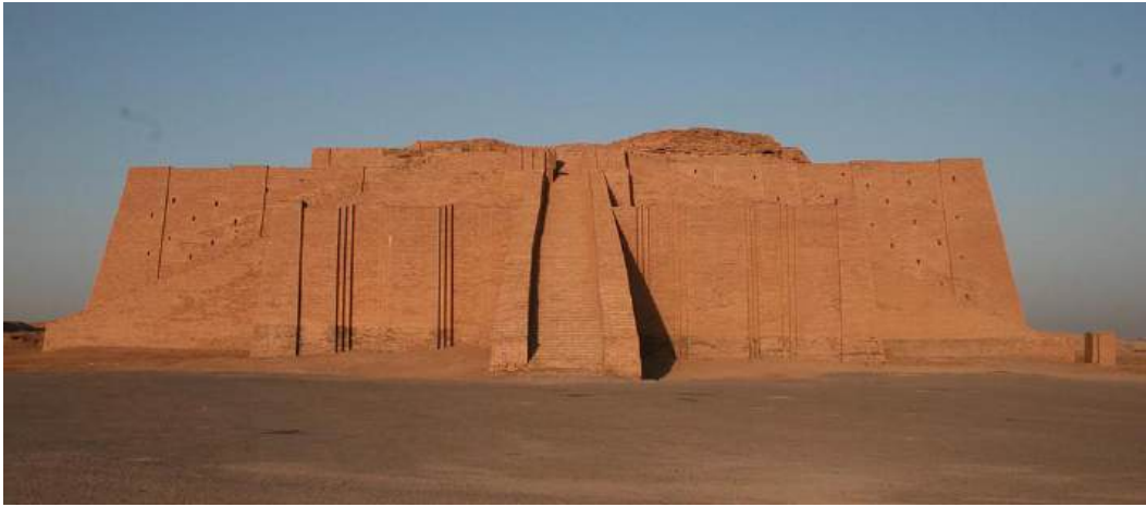
FIGURE 3.11 The Ziggurat of Ur. The partially reconstructed remains of the once-great ziggurat of Ur (near the modern city of Nasiriyah in Iraq) demonstrate the size of these huge temples and the enormous human resources spent on their construction. When it was completed in the twenty-first century BCE, this structure had additional tiers upon the large base shown and was about one hundred feet high. (credit: "Ziggurat of Ur" by "Tla2006"/Wikimedia Commons, Public Domain)
