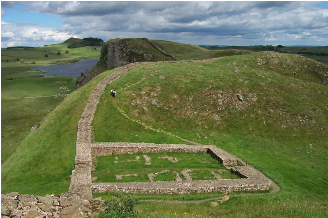
FIGURE 7.18 Hadrian's Wall. The massive Roman fortification built in Britain by the emperor Hadrian in the second century CE is roughly seventy-four miles long, with small forts known as milecastles placed at every mile along its entire length, as in the foreground of this photo. (credit: "Milecastle 39 on Hadrian's Wall" by Adam Cuerden/Wikimedia Commons, Public Domain)
