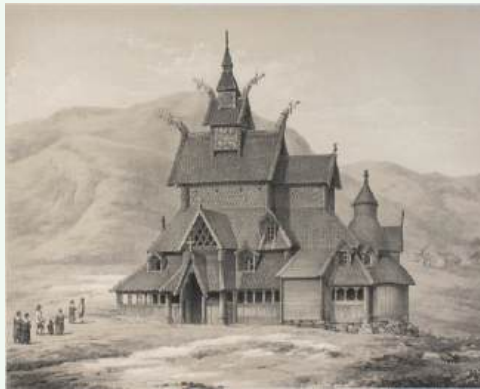
FIGURE 13.7 Borgund Stave Church. This nineteenth-century rendering of Borgund Stave Church was made by the Norwegian author Christian Tønberg. (credit: “Franz Wilhelm Schiertz Borgunds Kirke i Lærdal i Sogn” by Norge fremstillet i Tegninger fra Digitalarkivet/Wikimedia Commons, Public Domain)
