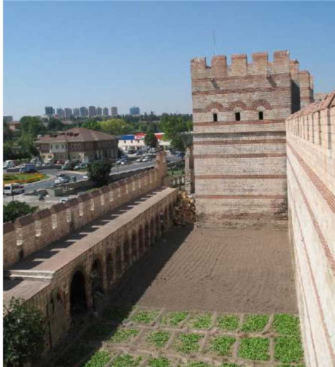
FIGURE 17.12 The Walls of Constantinople. The walls that protected Constantinople were massive. On the right is the inner wall, the city’s last defense. In places it was up to six meters thick. On the left is the outer wall. Below this was yet a third wall, and beyond that a moat. (credit: modification of work “Theodosian Walls in Constantinople” by “CrniBombarder!!!”/Wikimedia Commons, Public Domain)
