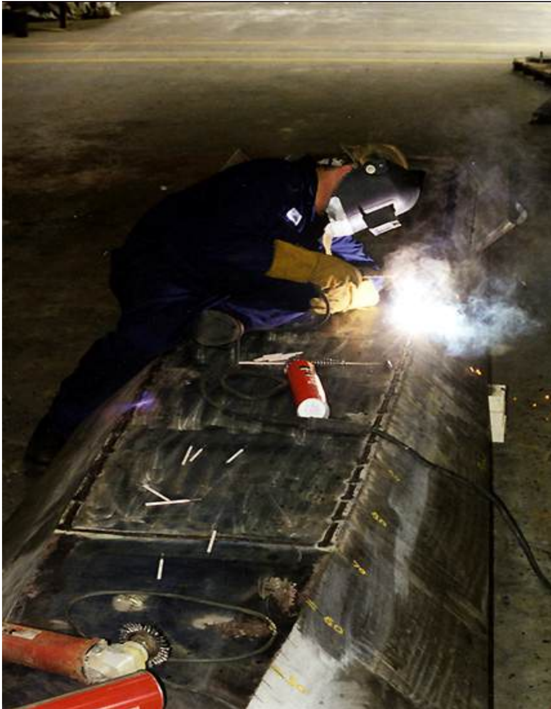
Photo 1: Stick Welding a Large Hopper
