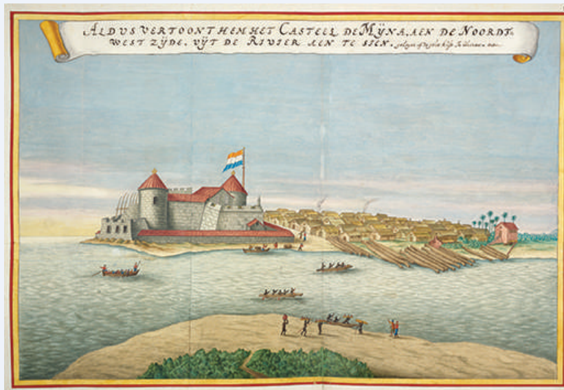
FIGURE 2.3 Elmina Castle on the west coast of Ghana was used as a holding pen for captured people before they were brought across the Atlantic and sold. Originally built by the Portuguese in the fifteenth century, it appears in this image as it was in the 1660s, after being seized by Dutch slave traders in 1637.
