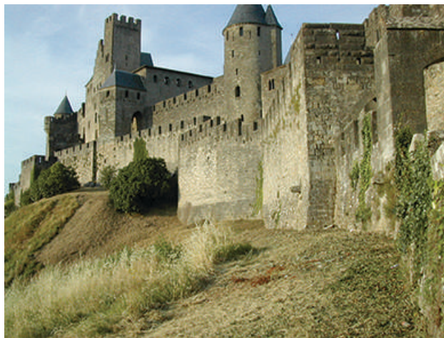
FIGURE 1.13 One of the most beautifully preserved medieval walled cities is Carcassonne, France. Notice the use of a double wall.
