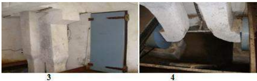
Showing the outer part of a bulk pasteurization chamber with its door closed and air handling unit (3) and the blowers fitted outside the pasteurization chamber
