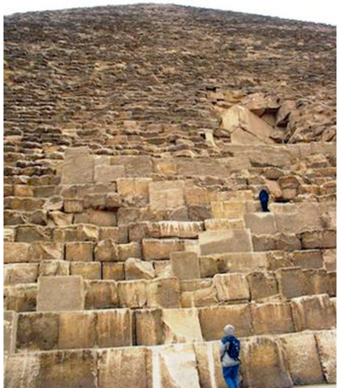
View up the side of Khufu's pyramid showing scale of the core blocks (Photo: Dr. Amy Calvert)
