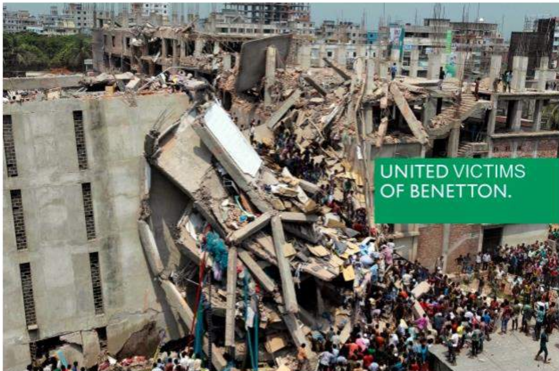
Image 13. Benetton faced reputation disaster when Rana Plaza collapsed.
