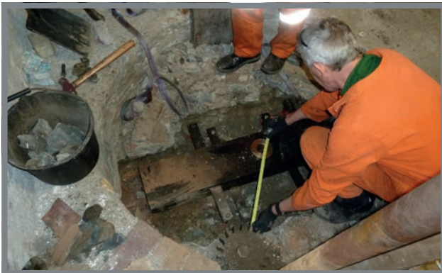
Positioning the new bearing and greasing system.
