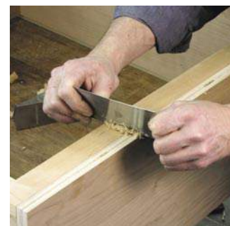
A card scraper brings the solid wood even with the plywood without raising a cloud of dust, or risking the damage that a belt sander or random-orbit sander could cause.
