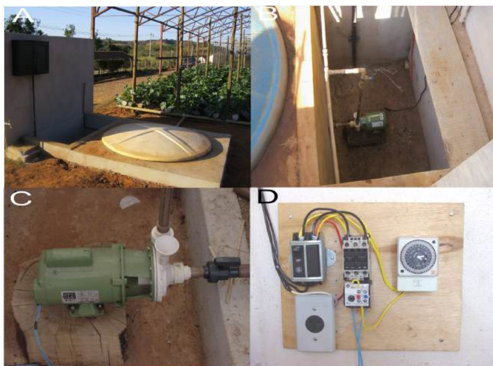
Fig. 2. Detail of the pump house (under construction) illustrating: A) Hydroponics being built by focusing the detail of water tank buried in the soil to avoid heating, B) and C) Set motor pump installed in a primed (below the level of reservoir), D) Panel containing outlet, timer relay and nutritious species. Photos: IFMG Bambuí, Professor Ricardo M. Corrêa.
