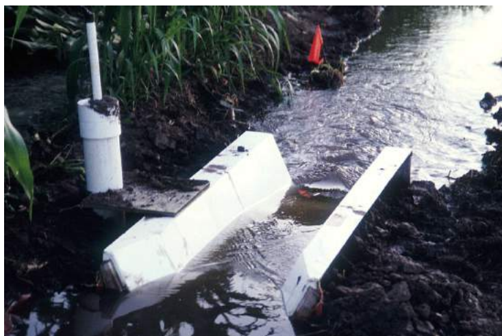
Figure 3.20. An RBC flume to measure open channel flow.
