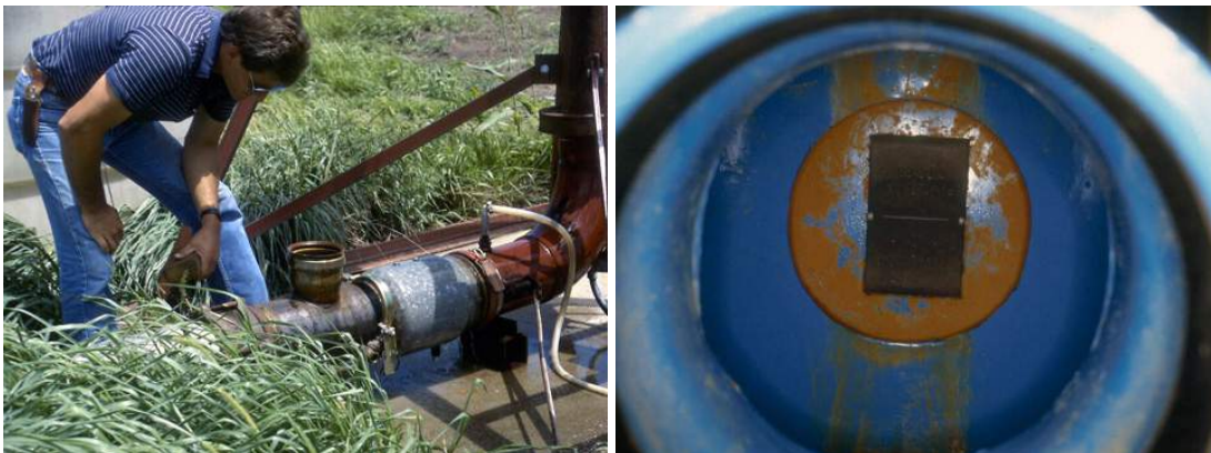
Figure 15.7. Inspection for check valve leakage in CCVA.
