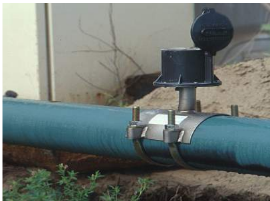
Figure 3.8. Field installation of a propeller meter.
