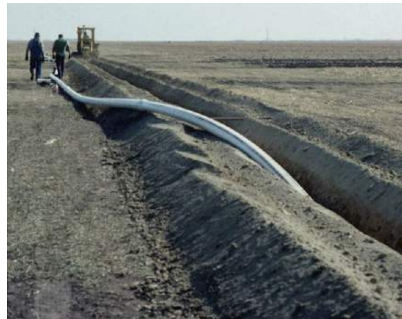
Figure 9.11. Installation of a buried pipeline for irrigation water delivery.
