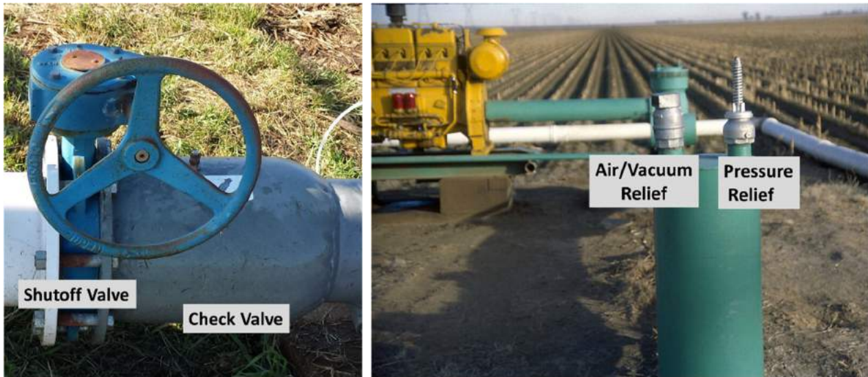
Figure 8.6. Irrigation pipeline protection valves.
