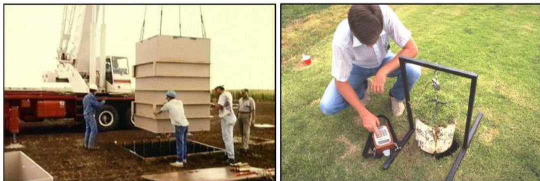
Installation of Large Precision-Weighing Lysimeter
