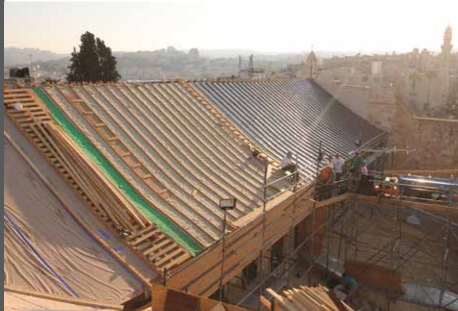
The roof of the basilica during the restorative works.
