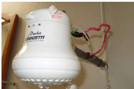
FIGURE 20.37 On-demand electric hot water heater. Heat is supplied to water only when needed. (credit: aviddavid, Flickr)
