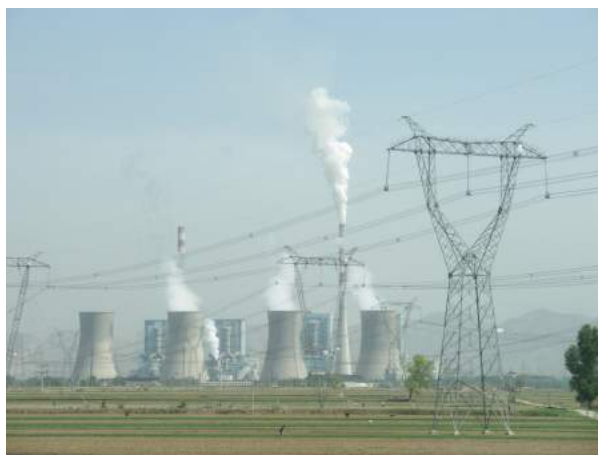
FIGURE 7.22 Tremendous amounts of electric power are generated by coal-fired power plants such as this one in China, but an even larger amount of power goes into heat transfer to the surroundings. The large cooling towers here are needed to transfer heat as rapidly as it is produced. The transfer of heat is not unique to coal plants but is an unavoidable consequence of generating electric power from any fuel—nuclear, coal, oil, natural gas, or the like. (credit: Kleinolive, Wikimedia Commons)
