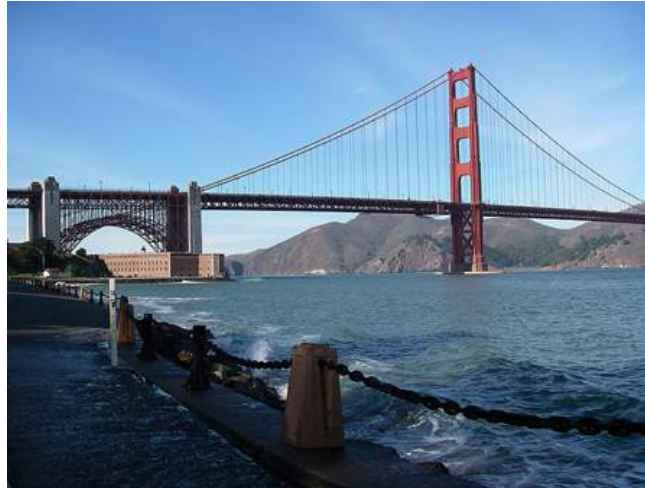
FIGURE 4.19 Unless an infinite tension is exerted, any flexible connector—such as the chain at the bottom of the picture—will sag under its own weight, giving a characteristic curve when the weight is evenly distributed along the length. Suspension bridges—such as the Golden Gate Bridge shown in this image—are essentially very heavy flexible connectors. The weight of the bridge is evenly distributed along the length of flexible connectors, usually cables, which take on the characteristic shape. (credit: Leaflet, Wikimedia Commons)
