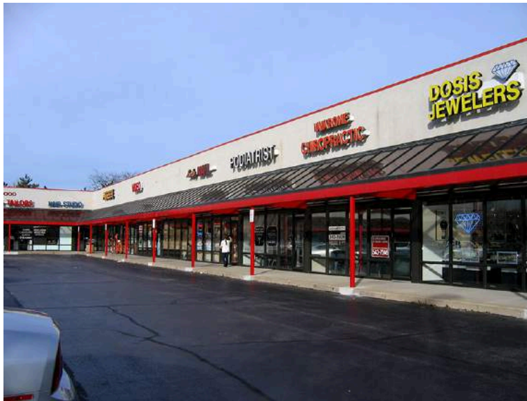
Figure 18.13 A strip mall is a collection of retail stores that consumers enter from outside the building. (credit: "20091112_001" by jarchie/flickr, CC BY 2.0)
