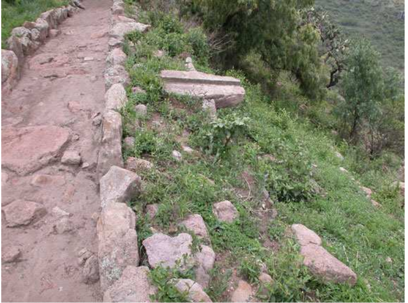
Figure 138. Circumambulation Path and Subsystem of Irrigation Canals (photo Fernando González y González).
