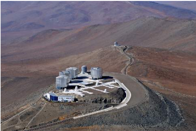
High and Dry Site - Figure 6. Cerro Paranal, a mountain summit 2.7 kilometers above sea level in Chile's Atacama Desert, is the site of the European Southern Observatory's Very Large Telescope. This photograph shows the four 8-meter telescope buildings on the site and vividly illustrates that astronomers prefer high, dry sites for their instruments. The 4.1-meter Visible and Infrared Survey Telescope for Astronomy (VISTA) can be seen in the distance on the next mountain peak. (credit: ESO)
