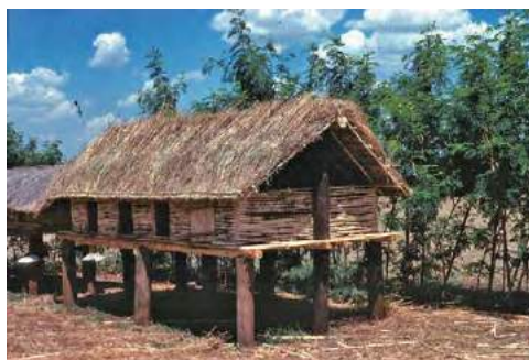
Fig. 4.6. A rabbitry in Malawi (East Africa) constructed of inexpensive local materials. Rabbits are quite suitable for small-scale production in developing countries. (Courtesy of J.I. McNitt)
