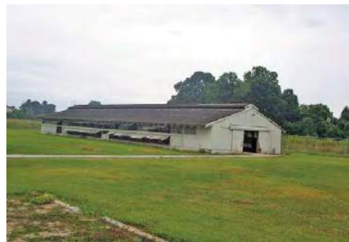
Fig. 4.1. A Louisiana rabbitry with side flaps that can be closed during inclement weather. (Courtesy of J.I. McNitt)
