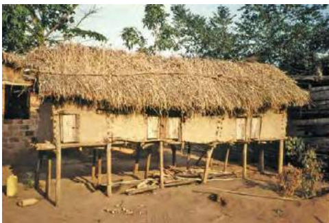
Fig. 1.4. A village rabbitry constructed of bamboo, palm thatch, and other locally available material. Rabbit production has considerable potential in developing countries. (Courtesy of S.D. Lukefahr)
