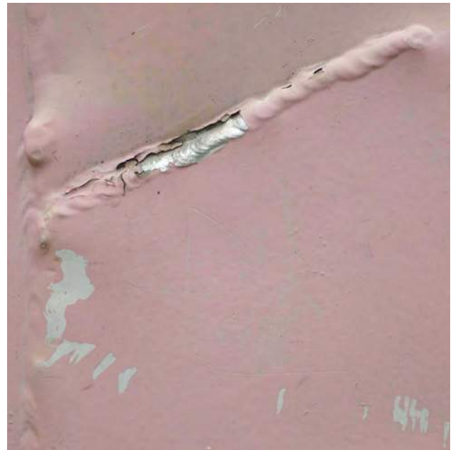
Figure 4 Detail of Flause , showing flaking paint caused by expansion of the aluminum underneath.
