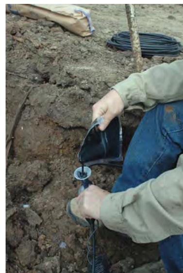
Figure 10c The cable connection housing is filled with a bituminous material to make the cable connections waterproof.
