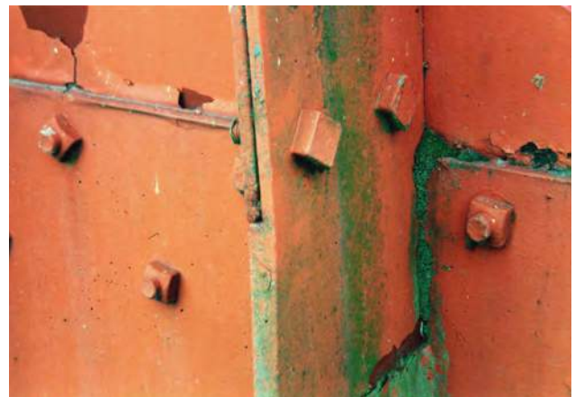
Figure 5 Photo of the west-facing side of Le Hallebardier , showing algae growth. © 2014 Calder Foundation, New York/Artists Rights Society (ARS), New York. © ZMK, Hannover 2003.
