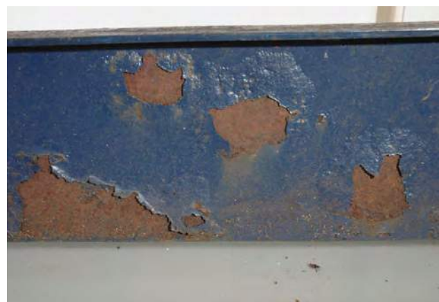
Figure 2 Detail of One for Bristol , indicating paint loss and corrosion in 2010. © The Artist's estate.
