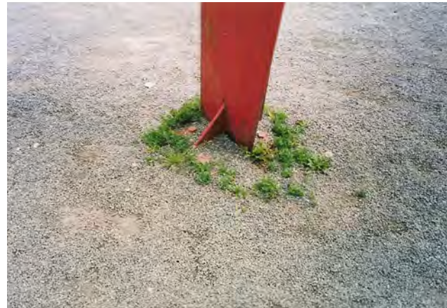
Figure 8 Corrosion damage is evident on the feet of the sculpture, caused by gravel with grass growing over the base plates. © 2014 Calder Foundation, New York / Artists Rights Society (ARS), New York. © ZMK, Hannover 2003.
