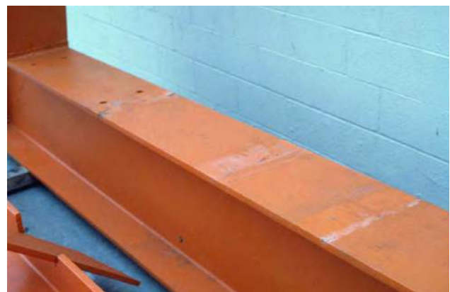
Figure 8 Detail of Rumi , showing abrasions caused by the straps used to secure the sculpture during shipping from the Di Suvero studio to the Nelson-Atkins Museum in 1995.
