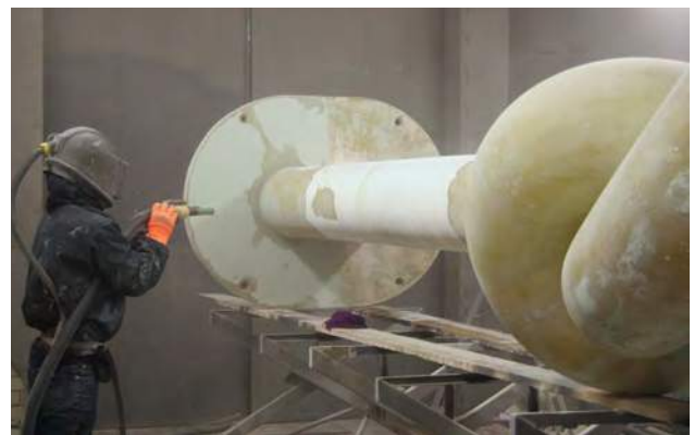
Figure 7 Sandblasting was used to remove the old paint layers. Photo: Lydia Beerkens.
