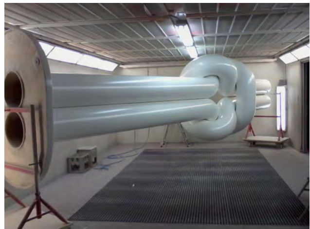
Figure 10 Square Knot in the spraying booth after applying the new white coating. Photo: Cees van Rijen.
