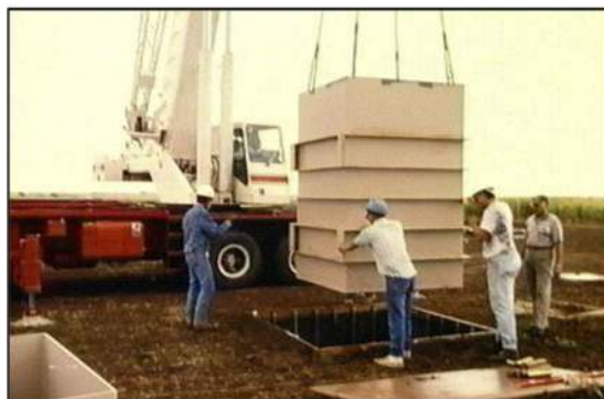
Installation of Large Precision-Weighting Lysimeter
