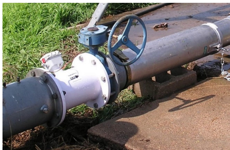
Figure 3.15. Electromagnetic flowmeter installed in the field.
