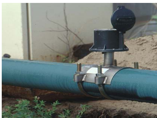
Figure 3.8. Field installation of a propeller meter.
