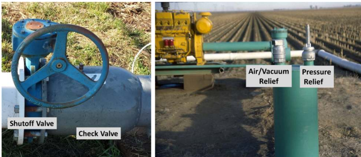
Figure 8.6. Irrigation pipeline protection valves.
