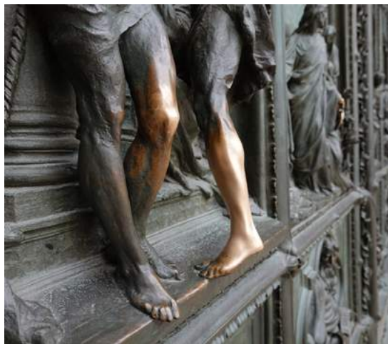
Fig.10/22 Constant visitor contact prevented the development of patina, revealing the true color of bronze.
