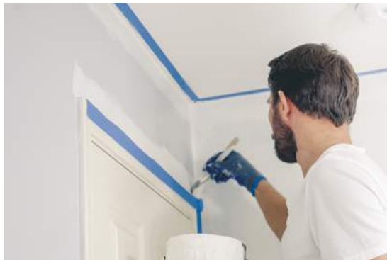
Fig.05/16 Painting is a messy process, and masking is a requirement for even the smallest job.
