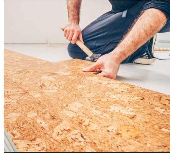
Fig.11/32 Cork is categorized as resilient flooring, though it cannot perform as well as polymers alternatives.
