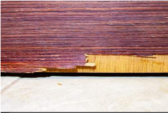
Fig.07/38 Veneer applications can check and peel over time, when exposed to moisture and abrasion.
