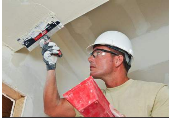
Fig.05/15 Skim coating involves a continuous layer of joint compound over finished drywall application.
