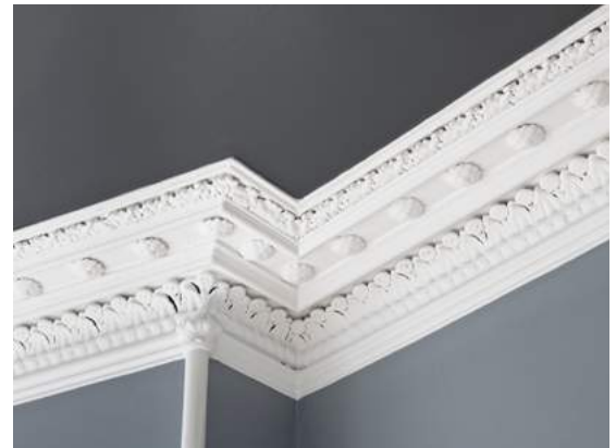
Fig.05/14 With silicone molds, plaster trims can feature highly intricate detail at a reasonable cost.
