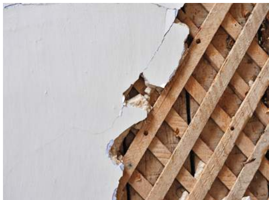
Fig.05/11 Plaster application over cross wood lath can still be found in some older housing.
