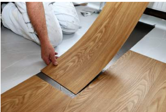
Fig.11/13 Luxury vinyl tile (LVT) can imitate any material thanks to a printable layer.
