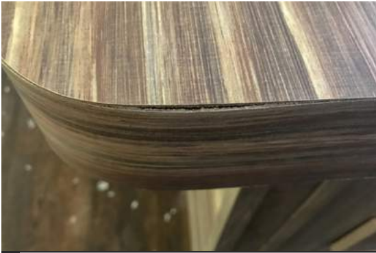
Fig.11/36 Plastic laminate edges and seams are prone to heat and moisture damage.
