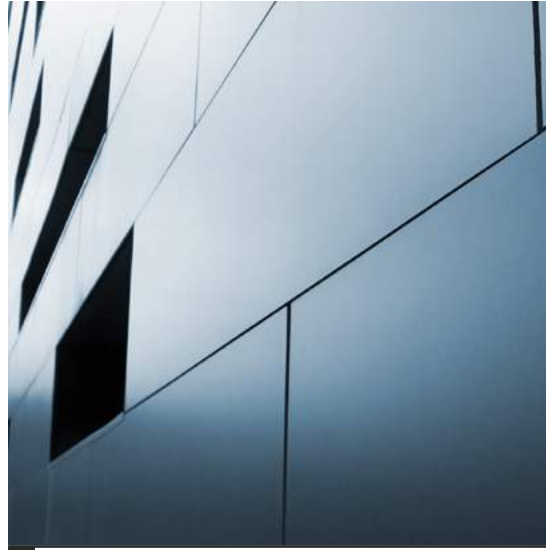
Fig.10/26 Zinc panels are commonly utilized in contemporary architectural facades.
