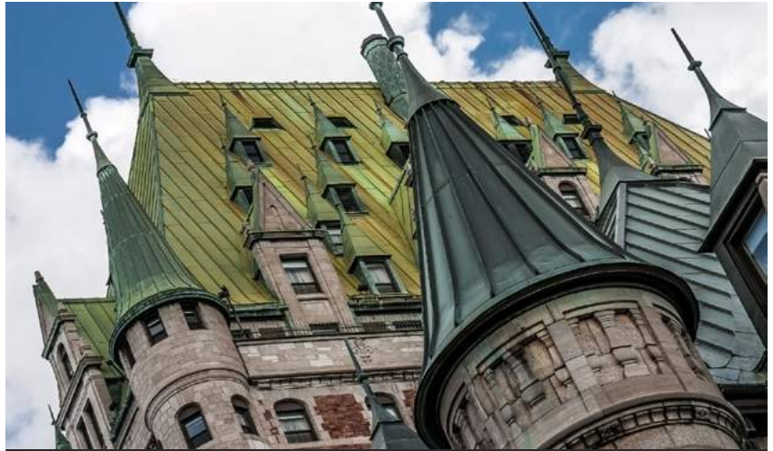
Fig.01/14 Every naturally developed patina features a unique look based on its location and surroundings.
