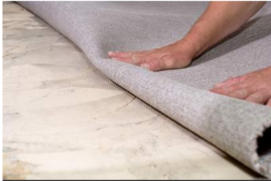
Fig.09/33 Glue-down application involves a thin layer of adhesive on a smooth substrate.
