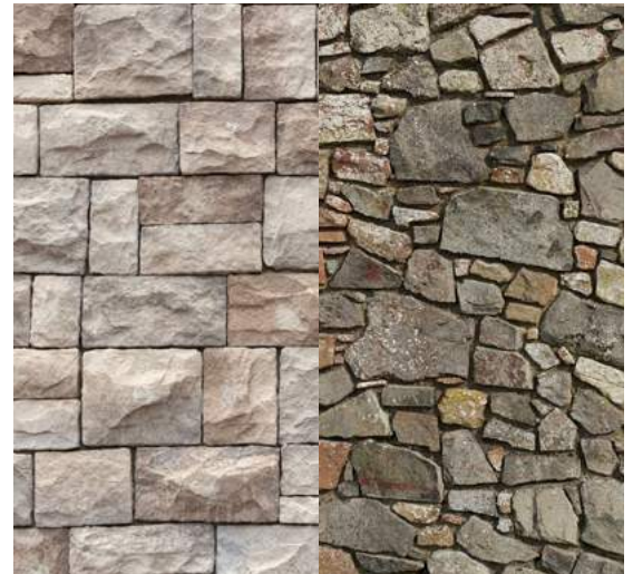
Fig.06/24 Ashlar masonry (left) is a stark visual contrast against rubble masonry (right).
