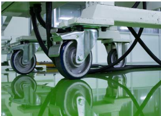
Fig.11/21 Epoxy flooring is actually a thin resin layer and requires meticulous substrate preparation.
