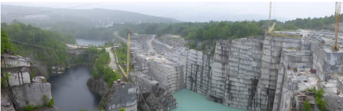
Fig.06/19 The Rock of Ages granite quarry is located in Vermont. It is the largest deep-hole quarrying operation in the world, measuring at 600 feet.
