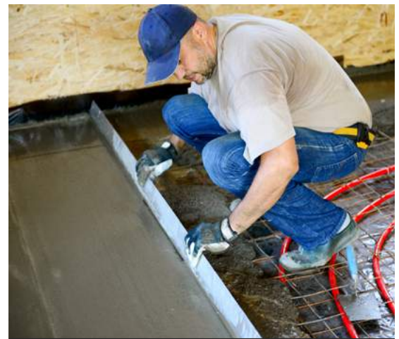
Fig.06/05 The screed is a flat board used to straighten freshly poured concrete.
