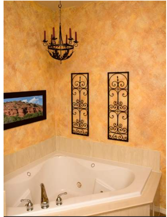
Fig.05/17 Textured paints are often applied with specialized or unusual tools, requiring a lot of skill.
