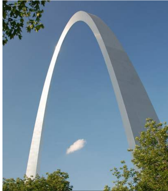
Fig.10/02 304 series stainless steel alloy panels were used for the Gateway Arch construction.
