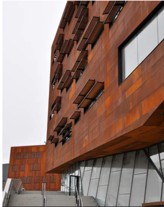
Fig.10/18 Weathering steel panels introduce unique earthy colors and natural texture variations.
