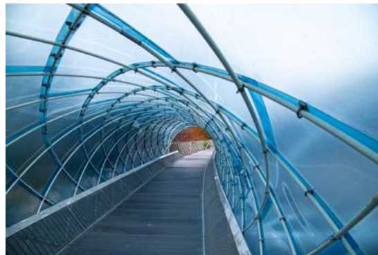
Fig.08/05 Glass panels can be bend bi-directionally and tempered to cover curved public walkways.
