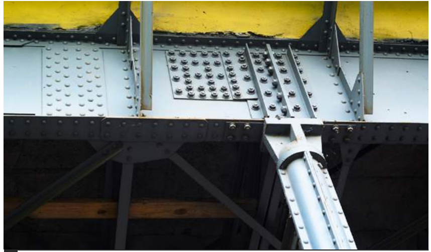
Fig.10/08 Riveting is a time consuming process, harder to conduct on-site, therefore a mixture of rivets and bolts is not an uncommon sight in construction.
