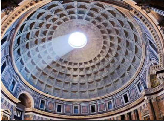
Fig.06/01 The dome of Pantheon showcases the capabilities of concrete as a construction material.
