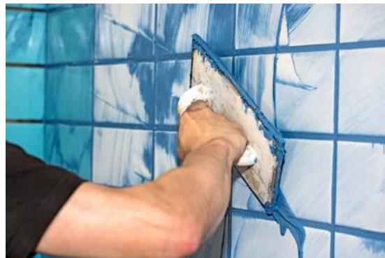
Fig.08/25 Without the use of grout release, colored grout applications can easily stain white tiles.
