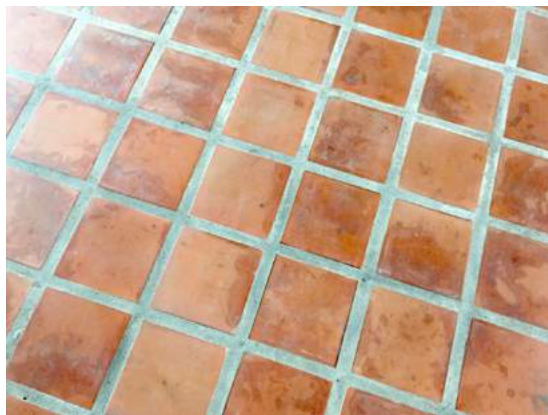
Fig.08/19 Contrary to what their name suggest, quarry tiles are actually fired clay.
