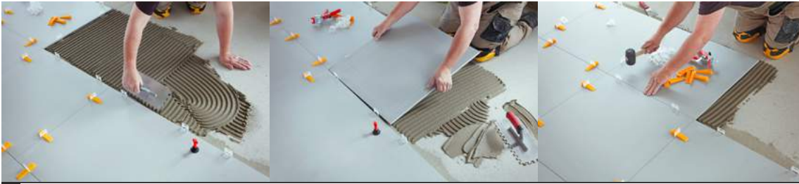
Fig.08/23 The three steps for tile installation: troweling, laying, and compressing.
