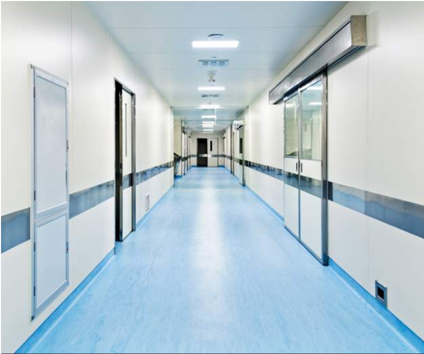
Fig.11/11 Vinyl flooring application in an operation room corridor, the welded seams and flash coving at the perimeter are compatible with the strict hygiene require-
