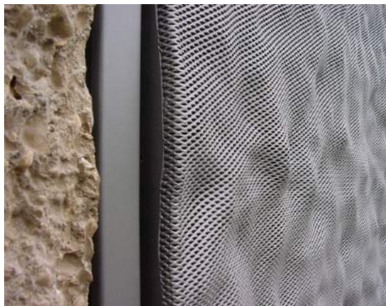
Fig.09/11 A non-woven metal sheet product, expanded metal mesh is able to hold form.
