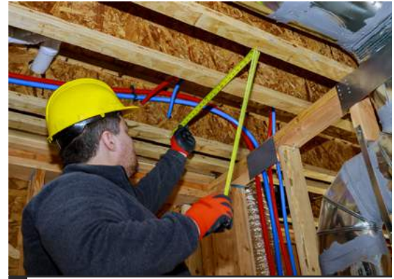
Fig.11/09 Thanks to their flexibility, PEX pipes can be run like electrical conduits, without elbow joints.
