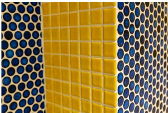
Fig.08/24 Mosaics feature a much higher grouted area compared to other tile types.
