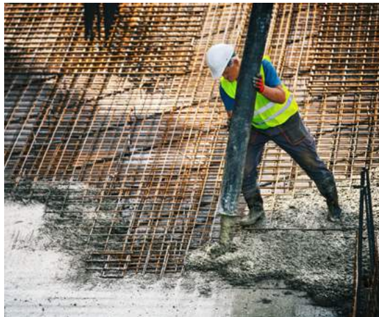
Fig.01/11 Concrete mixture poured over rebar lattice.
