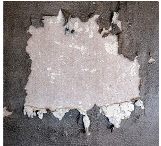
Fig.09/20 Artificial leather is highly susceptible to cracking and peeling.
