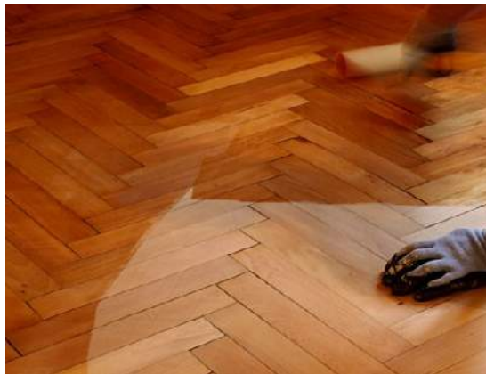
Fig.03/10 Polyurethane topcoat emits VOCs intensely for 4 days, and with decreasing intensity for up to 30 days.
