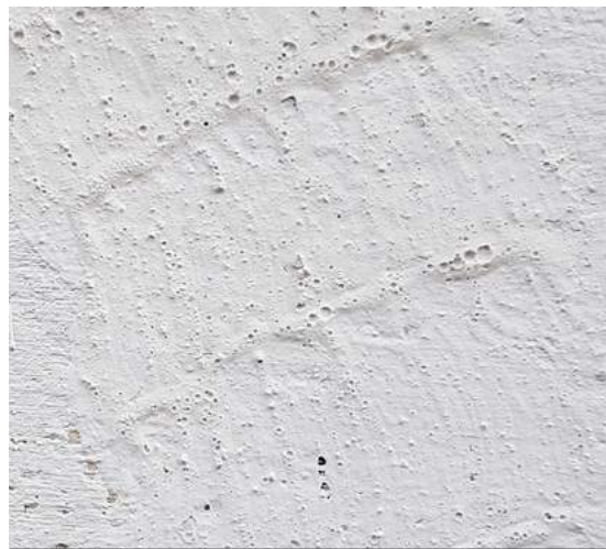
Fig.05/03 In order to mitigate the tiny craters, defoaming agents should be mixed in the paint formula.
