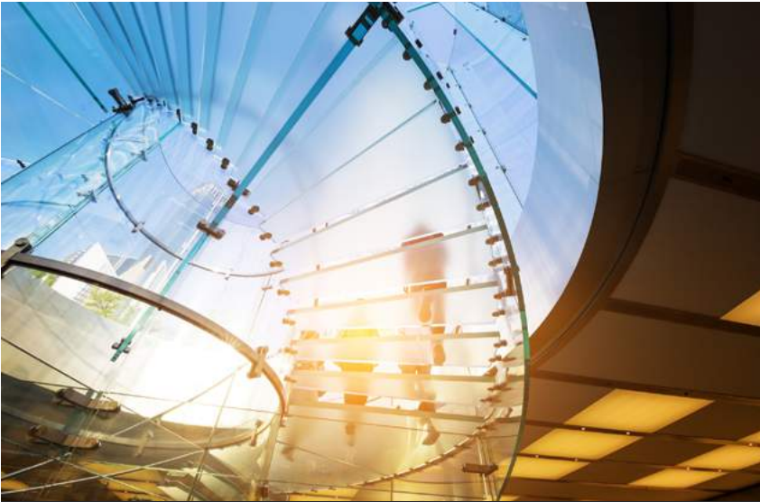
Fig.08/06 It is possible to use laminated glass as load bearing member in less structurally demanding situations such as supporting stairs.
