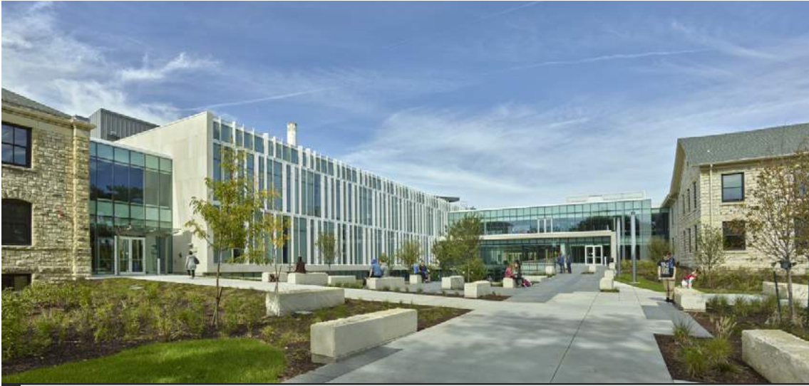
Fig.04/10 The KSU College of Architecture, Planning and Design is housed in the LEED Silver certified Seaton Hall.
