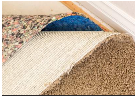
Fig.09/29 Carpet pads improve both physical and acoustical performance of the carpet.
