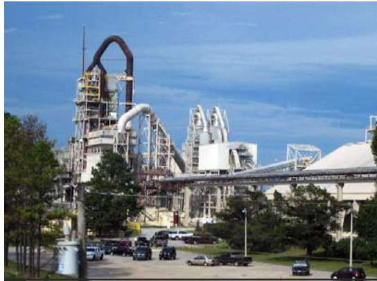
Fig.06/02 Portland cement factory. The long tube diagonally running left to right is the kiln.
