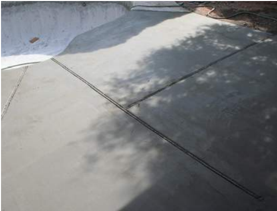
Fig.06/06 Expansion joints are crucial for protecting the integrity of the concrete for extended periods.
