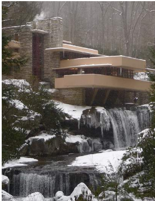
Fig.02/04 The concrete cantilevers in Fallingwater House sets a stark contrast with nature.
