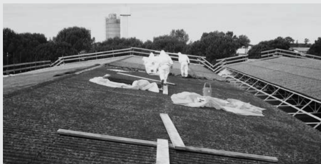
Asbestos removal
