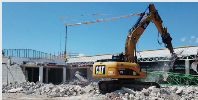
Demolition of old premises
