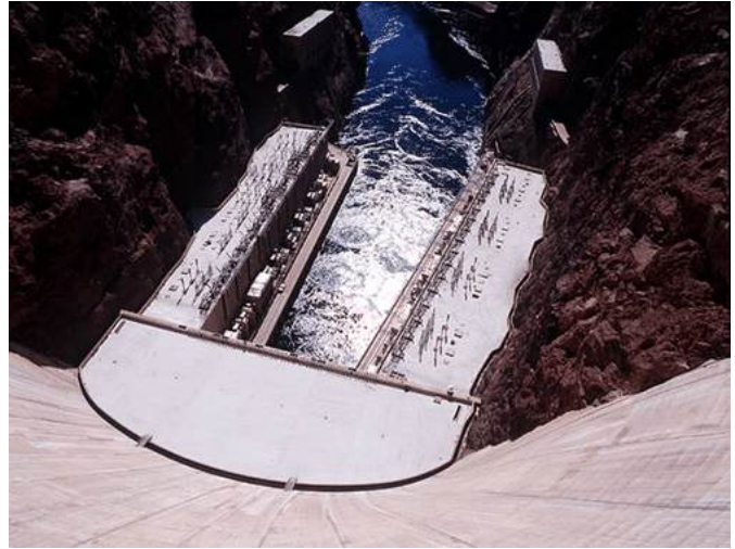
Figure 1. Hoover Power Plant View of Hoover Power Plant on the Colorado River as seen from above. Source: U.S. Department of the Interior
