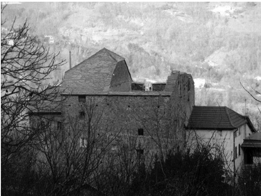
Fig. 1 & 2 Medieval building around Genoa, partially uncovered.
