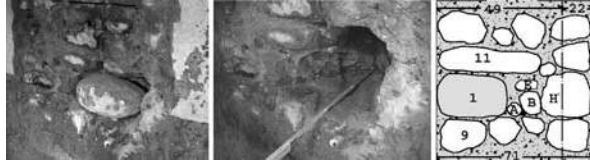
Figure 8 Study of the masonry morphology on a Church in Brescia province.
