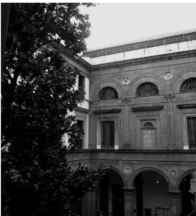
Fig. 2 Naples, Gravina Palace. Detail of the courtyard, surrounded by piperno arches and pillars.
