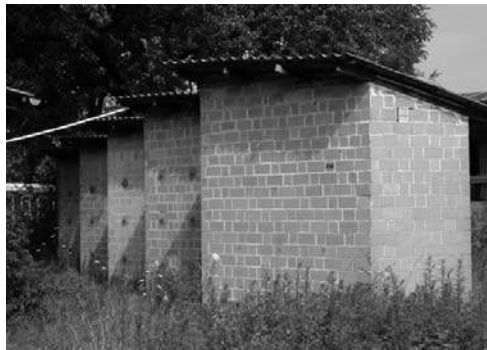
Figure 10 Masonry prototypes subjected to natural and accelerated damage.
