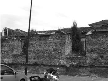
Fig. 7 The outside wall rests of the Quartiere di Cavalleria measured and widened by Colonel Barabino in 1832.
