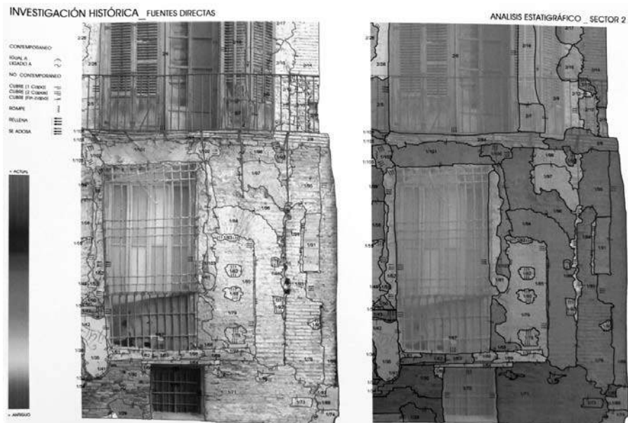
Fig. 3 Example of a stratigraphic analysis of a facade made by a group of graduate course students.
