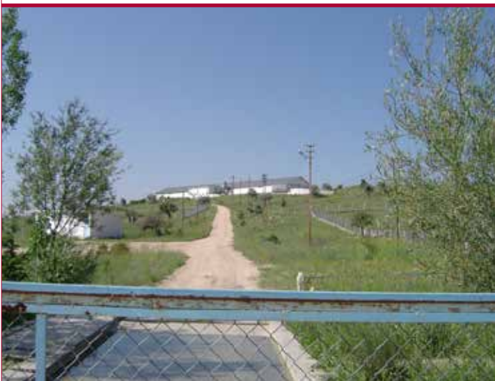
This poultry facility has good topography for rain drainage away from the building, utilities, fencing for bio-security, and appears to be located away from nearby residents – all good siting practices.
